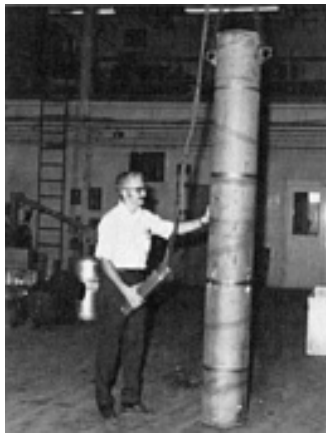
Fig. 20 Large-sized cylindrical high-speed steel billet. Courtesy of Crucible Materials Research Center
